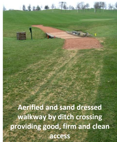
Aerified and sand dressed walkway by ditch crossing providing good, firm and clean access
