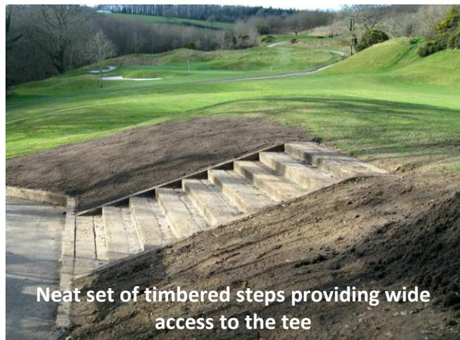
Neat set of timbered steps providing wide access to the tee
