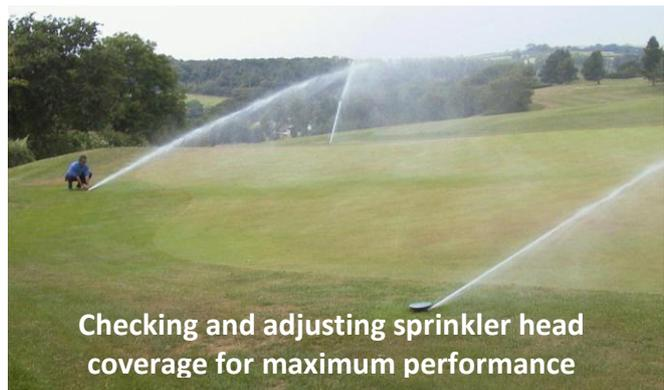
Checking and adjusting sprinkler head coverage for maximum performance
